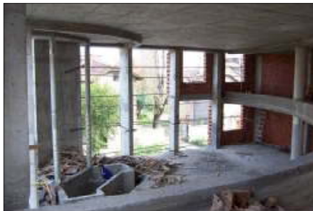
The Conference Facility under construction
