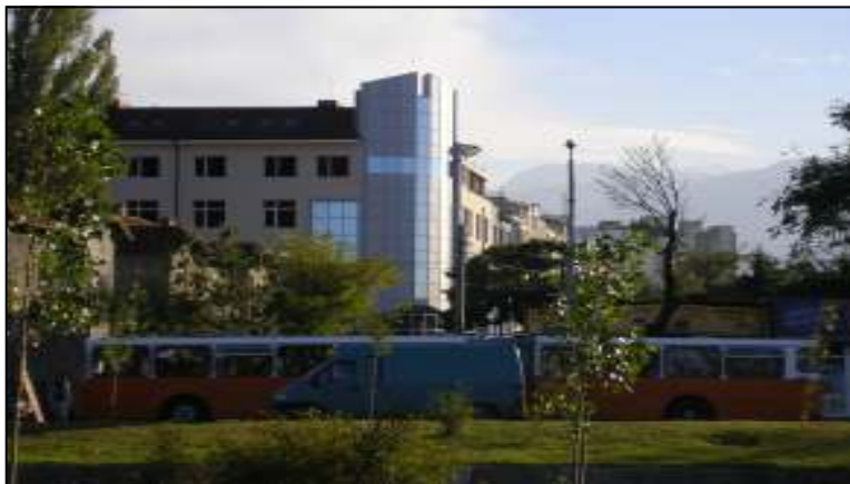
The Sofia Church Community Training Centre under construction
